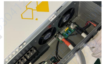
Inverter positive and negative pole installation completed status
