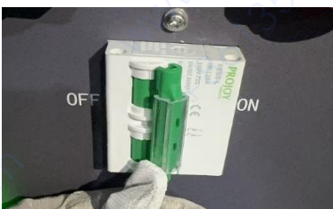
Turn on the battery main switch
