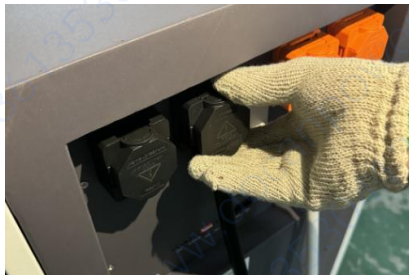
Cover the negative electrode with a protective cover after assembly
