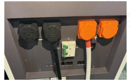
Battery positive and negative pole installation completed status
